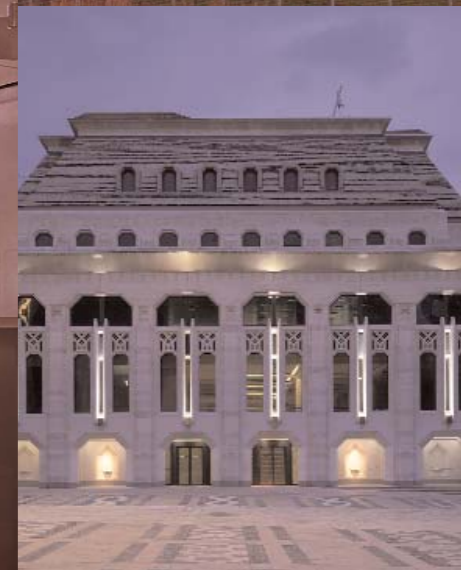
Left and above - Guildhall in London protected by Sapa Powerframe system. Top right - buildings around fuel depots can be vulnerable
